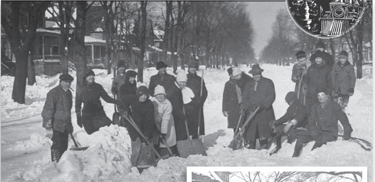
January 1918 blizzard; 4100 block of Keeler looking north
